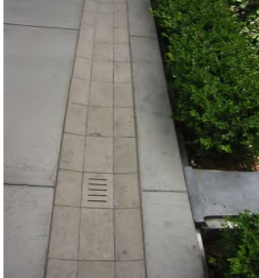
Constructed swale with drain (Credit: Stephanie Landregan)
