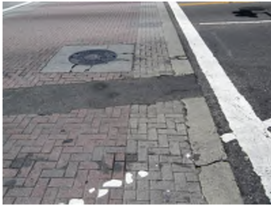
Decorative crosswalk treatments made of distinctive materials can become uneven over time. (Credit: Ryan Snyder)
