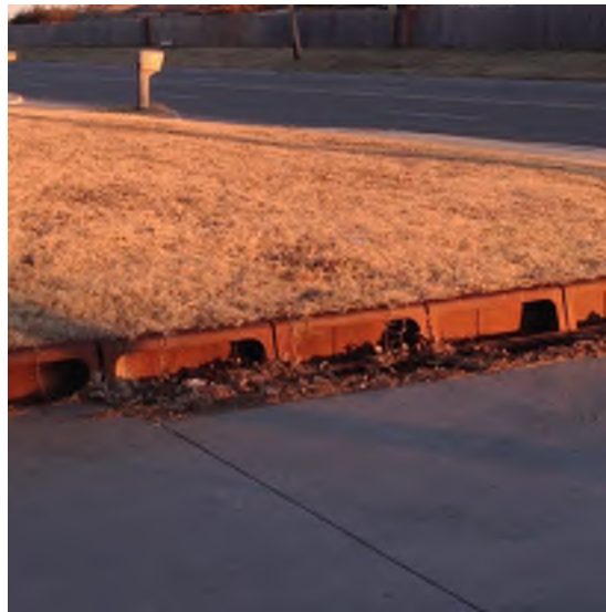
Curb inlet grate catching debris (Credit: David Riesland)
