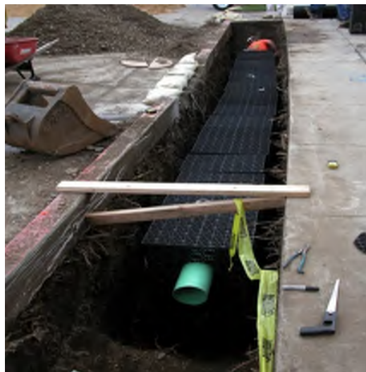
Infiltration trench with perforated pipe during installation (Credit: Neil Shapiro)
